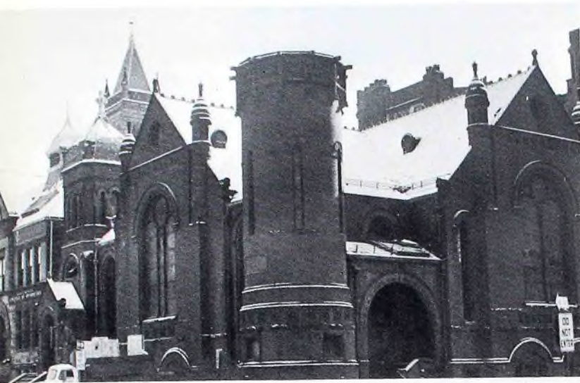
Before . . . Copley Methodist Church next to main building at 178 Newbury Street just prior to razing.
